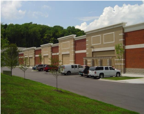
Figure 905-A: This figure shows two methods of using architectural features to create wall surface relief on wall elevations that are not the primary elevation.
