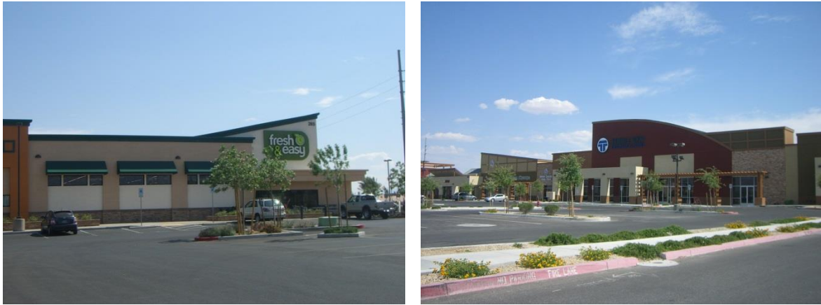
Figure 905-F: An example of dynamic roof lines
